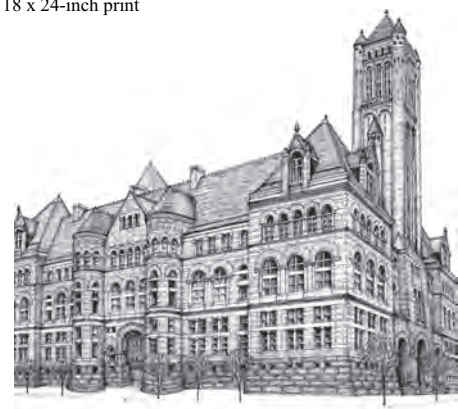
Allegheny County Courthouse
